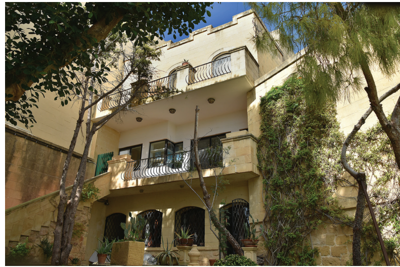
Back facade overlooking garden
