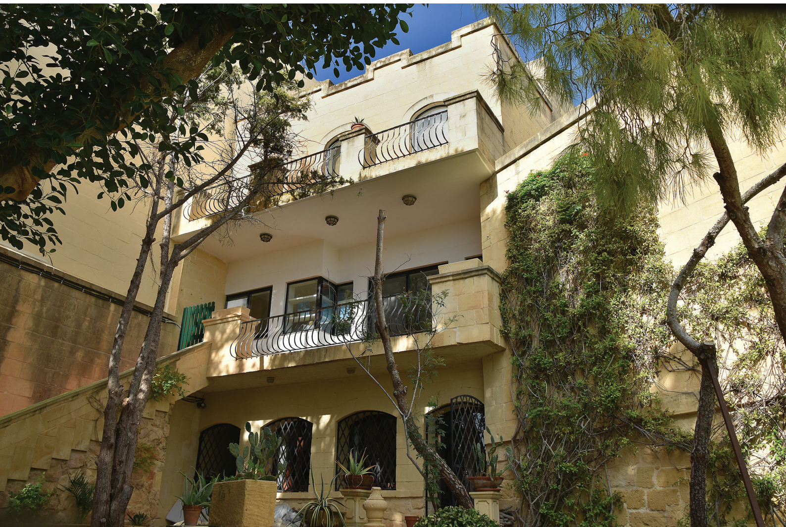
Back facade overlooking garden
